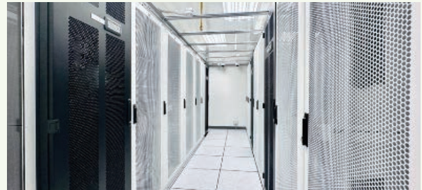
Using in-row air-conditioning system for energy saving and better cooling performance
